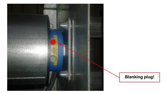
Photo 1. Curtain motor limit switches
